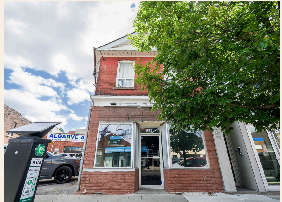
THE 3331 STOREFRONT AND PRIVATE ENTRY, SEEN FROM THE WEST
